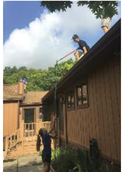
A few brave souls spent some time cleaning the gutters & putting on gutter screens.
